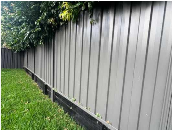
Termite and Timber Pest 4.03
