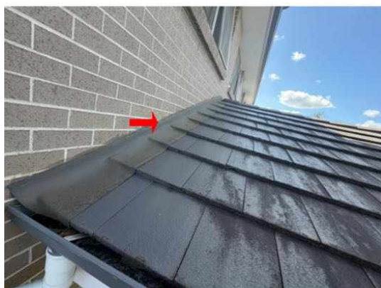
DIAGRAM 8.09 FLASHINGS
