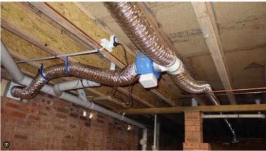
Sub-Floor Ventilation Kit with VEM 125 with BTU - Up to 70m2 $ 1,995.00 - $2795.00 - 10 items - Brand Universal Parts This sub-floor ventilation kit is designed to service areas up to 70m2. This sub-floor ventilation system features an 80mm VEM 125D Duct-Fuge Fan...
