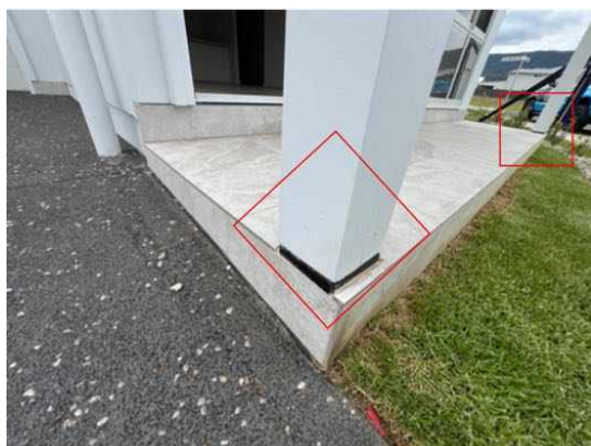
FIGURE 3.1(D) METAL STIRRUP AS ALTERNATIVE TO SHEETING FOR POSTS
