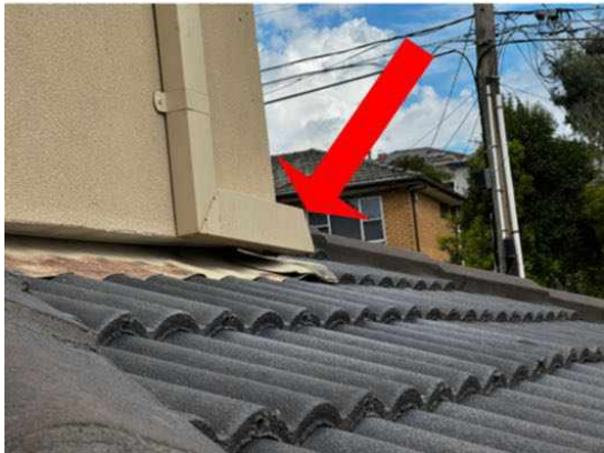
Non compliant roof discharge
