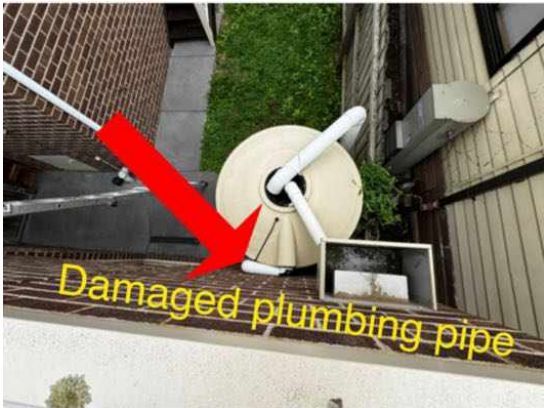
Discharging directly onto roof flashing
