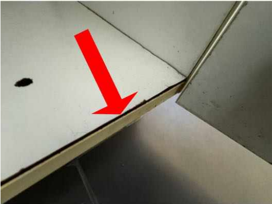
Moisture damage to laundry cabinets
