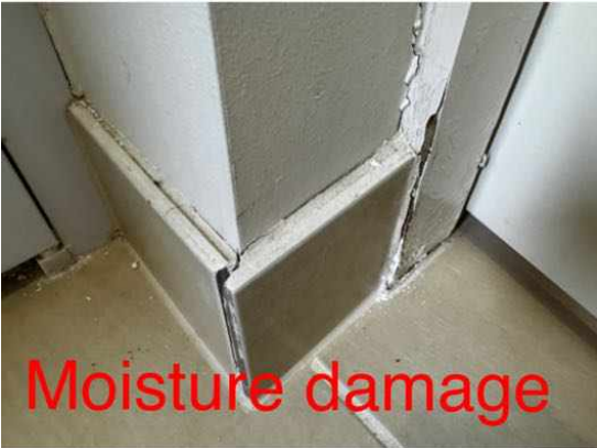
High moisture reading
